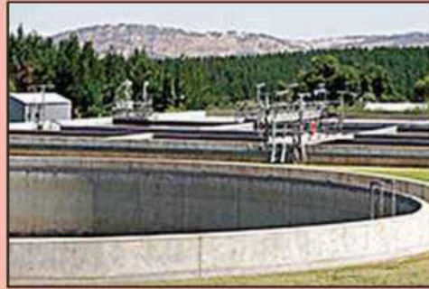
Fig: Sewage treatment plant.
